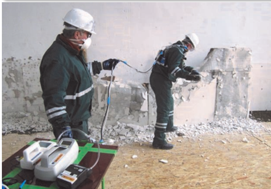
Figure 2: Workers in Romania and Poland performing various works involving materials with MNMs, with simultaneous measurement of the NP concentrations in air.
